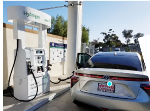
LH2 storage and dispensing for passenger cars
